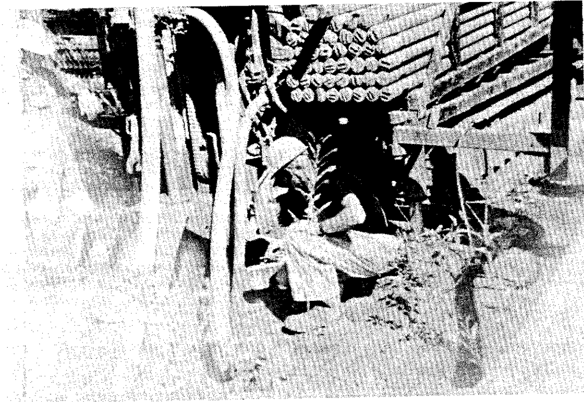
PHOTO 3 Checking the Ground for Blow-by Losses
