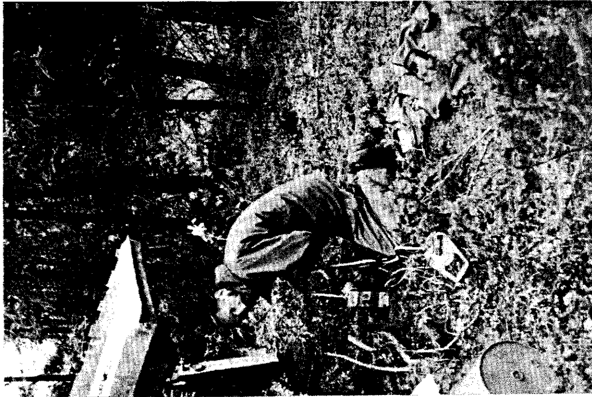
PHOTO 28 Lowering Scintillometer Down Auger Drill Hole
