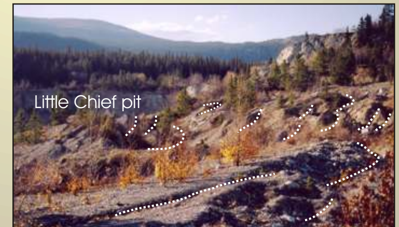
Right: slumping ground on east side of pit; dotted lines mark scarps.
