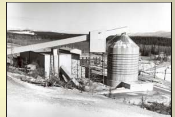
New Imperial Mines Ltd.: Surface buildings, circa 1970. The cylindrical tank was a storage bin for finely crushed ore.
