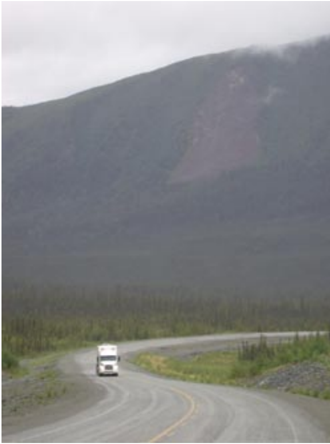
Figure 15. Looking east at Wolf Creek rock slide, Alaska Highway in foreground.
