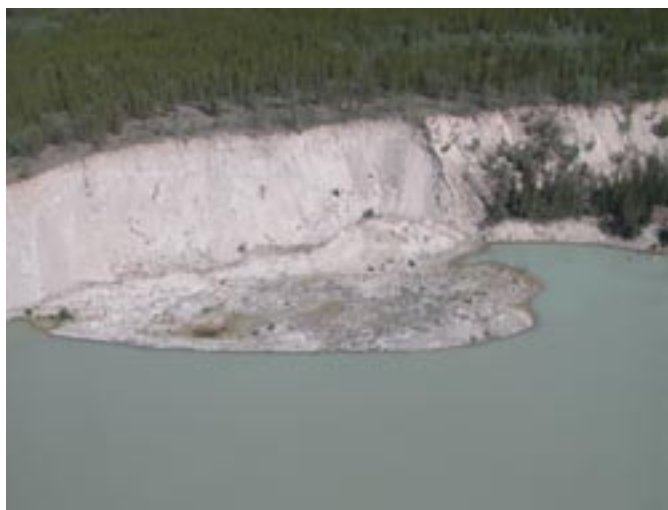
Figure 25. Earth slide due to river erosion and undercutting of glaciolacustrine silts in the Takhini Valley.
