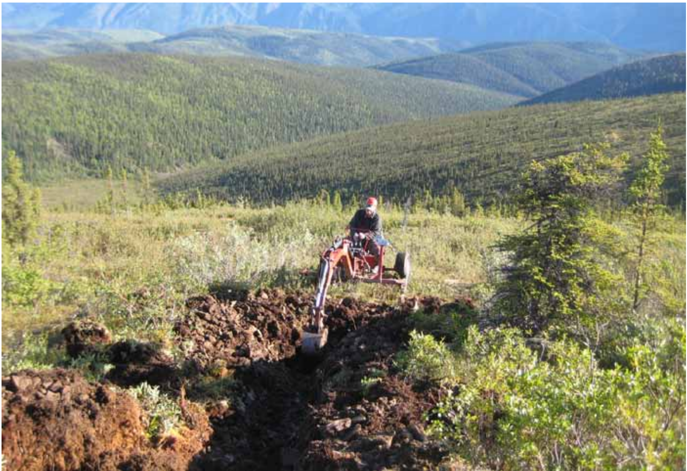
Figure 45. Trench excavation on a northeast-facing slope on the Coffee Property using a CanDig® Mini Excavator.
