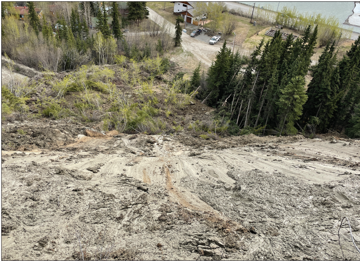
Figure 36. View looking down Drury Street slide from the headscarp (May 27, 2022 photo).
