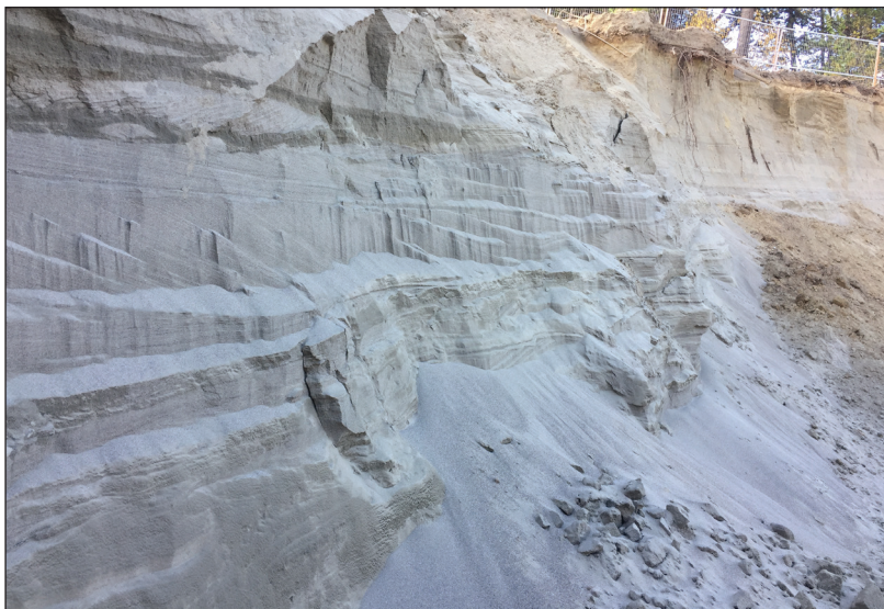
Figure 17. Approximately 5 m of well-sorted deltaic (glaciofluvial) sand exposed in a foundation excavation in the Takhini North subdivision (20PL038).
