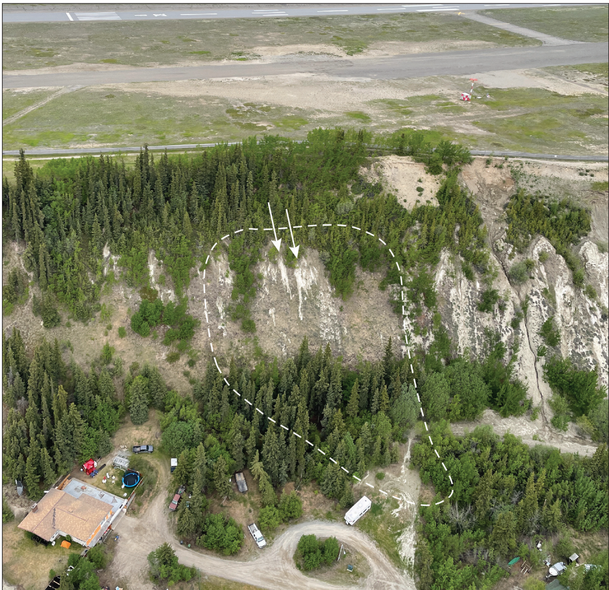
Figure 35. Drury Street slide area (outlined) prior to the May 25th, 2022 event (June 2021 photo). Arrows highlight recent colluvial activity in the initiation zone area.
