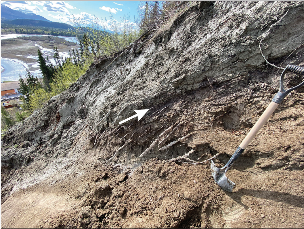
Figure 8. Fine-grained colluvium exposed on the Whitehorse escarpment on the south lateral margin of the 2022 Drury Street landslide initiation zone (J. Bond photo). Note buried organic horizon (arrow) and bedding structure parallel to the slope angle.
