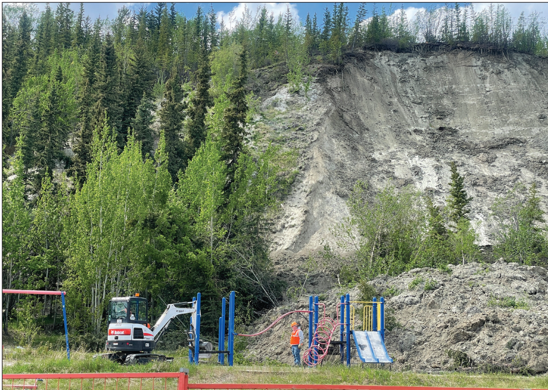
Figure 42. View of Jeckell Street slide debris, which engulfed a playground swing set. Initiation zone and failure plane are visible in the background.
