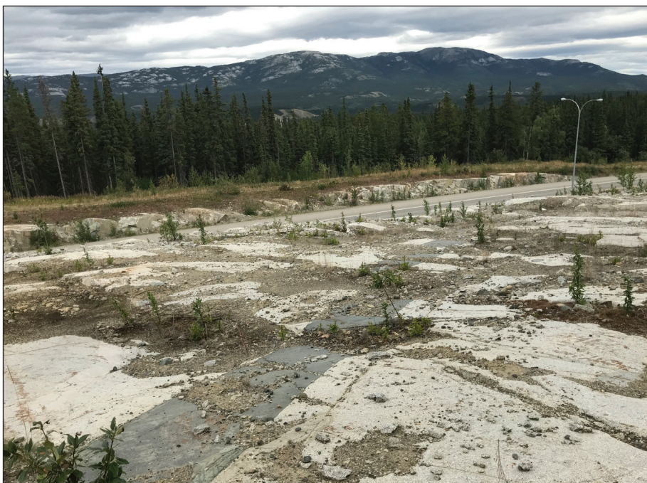
Figure 21. Scoured granodiorite with crosscutting dikes exposed after stripping thin overburden along the Hamilton Boulevard extension.
