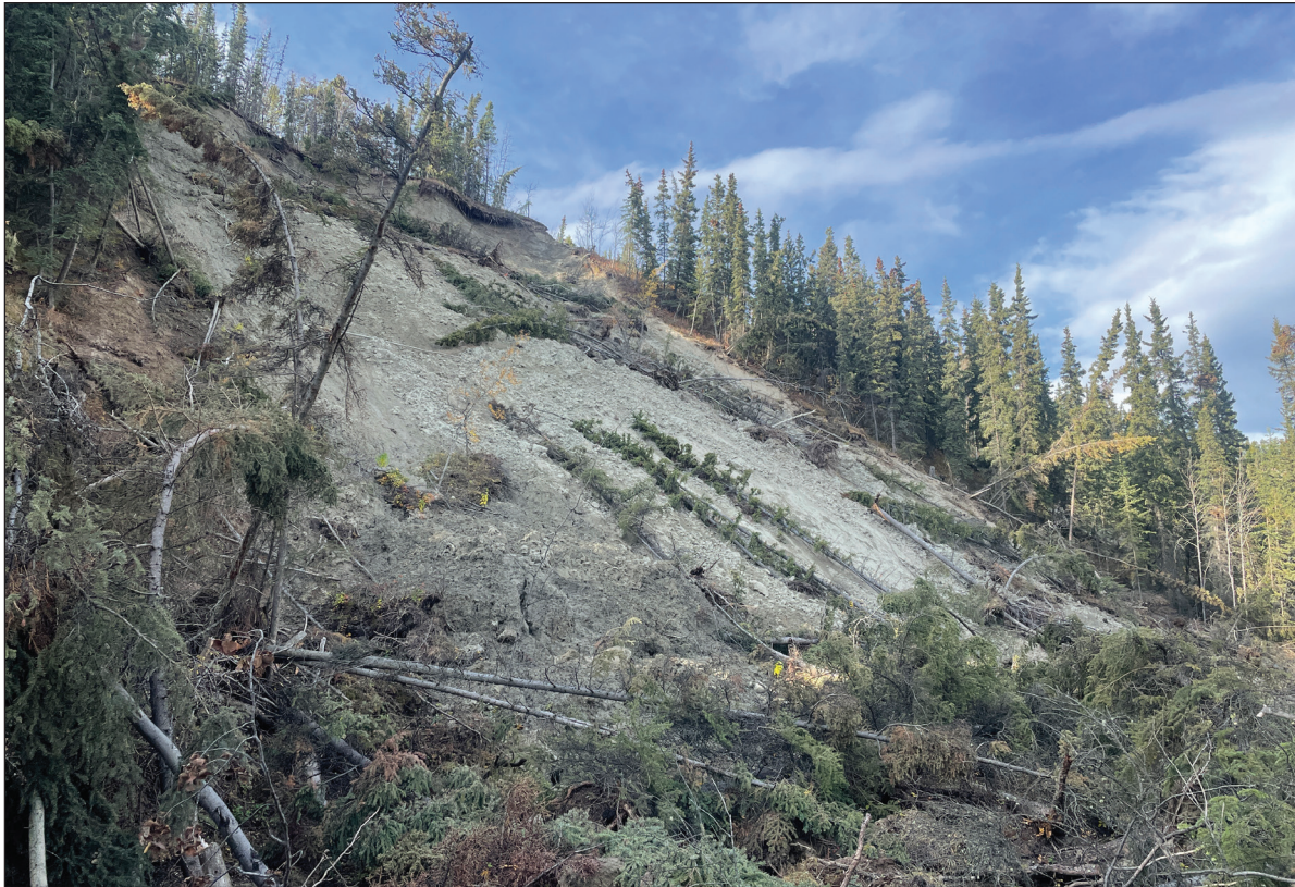
Figure 43. Initiation zone and failure plane of May 31, 2022 earth slide off Robert Service Way (October 10, 2022 photo).
