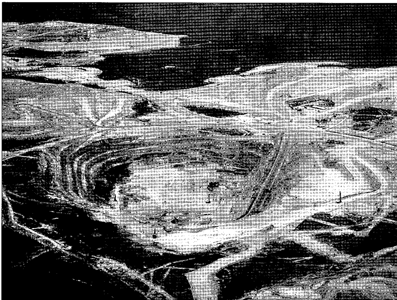
FIGURE 5: The Faro Lead-Zinc-Silver Mine of Anvil Range Mining Corporation reached full production from the Grum Pit in 1996. The mine reopened in August, 1995 after a two year closure. To the end of the third quarter Faro produced 151.2 million kg Zn, 90.9 million kg Pb and 153,000 kg Ag for a value of production of approximately $320 million.
