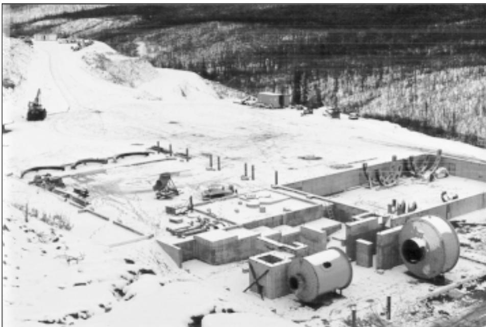
**Figure 6.** Assembly of the semi-autogenous grinding (SAG) and ball mills were completed in the fall of 1999 at the Minto project. The completed mills are ready for installation on the mill foundation. Photo by Minto Explorations Limited
