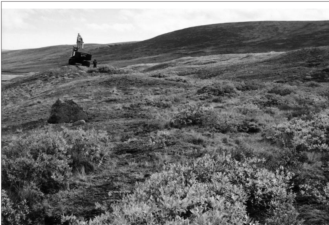
Figure 1. Walking a backhoe across the tundra to the Killer Gold property, Killerman Lake area.
