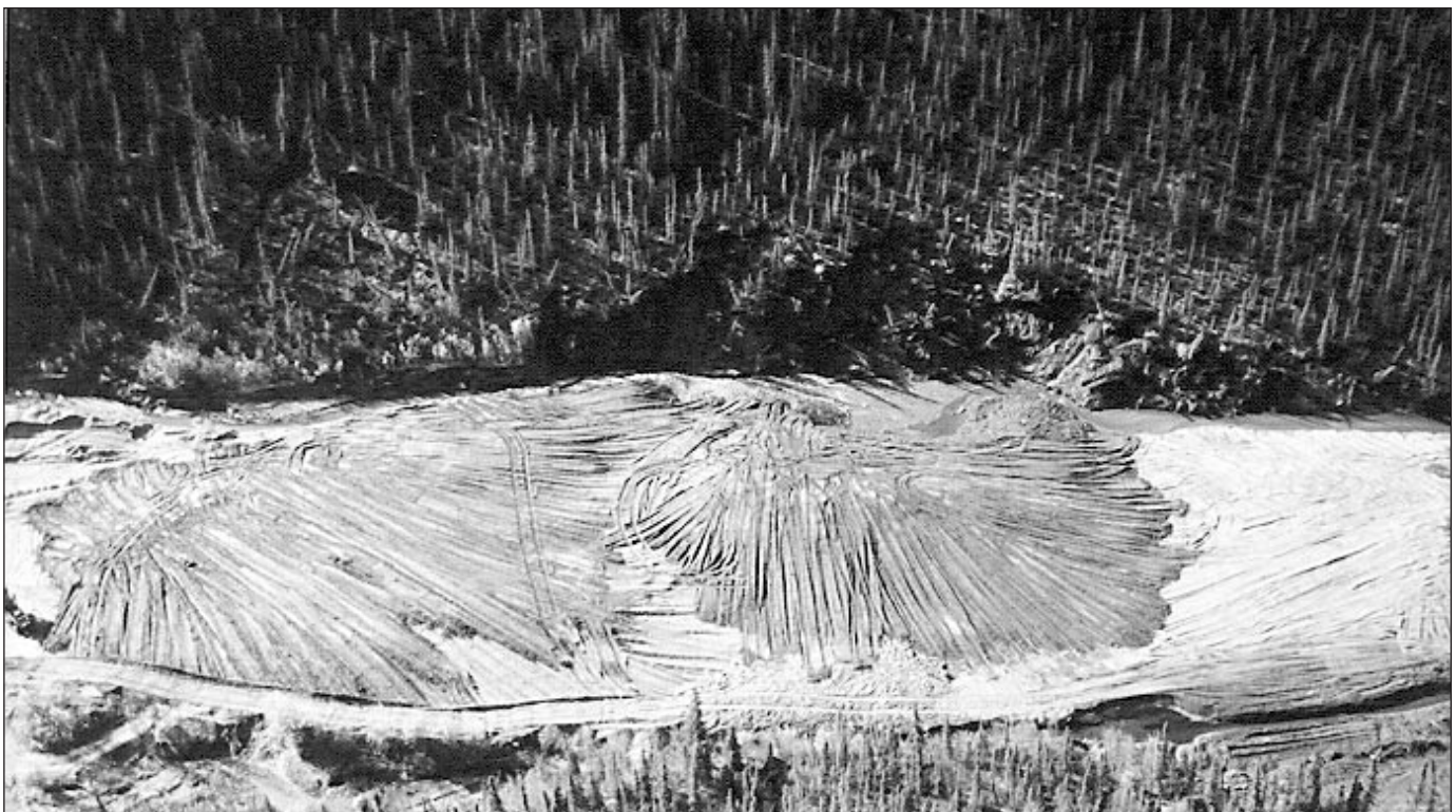
Figure 2. Contoured tailings at Hunker Creek are covered with 'black muck' to enhance natural revegetation.
