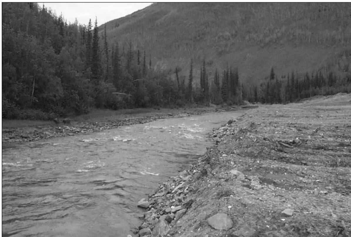
Figure 3. David McBurney's restored river bank, with large rock armouring along the bank and overburden spread up to the edge.
