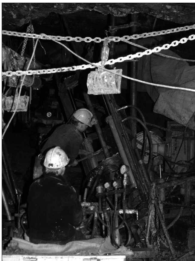
Figure 11. Underground drill at the Skukum Creek deposit.
