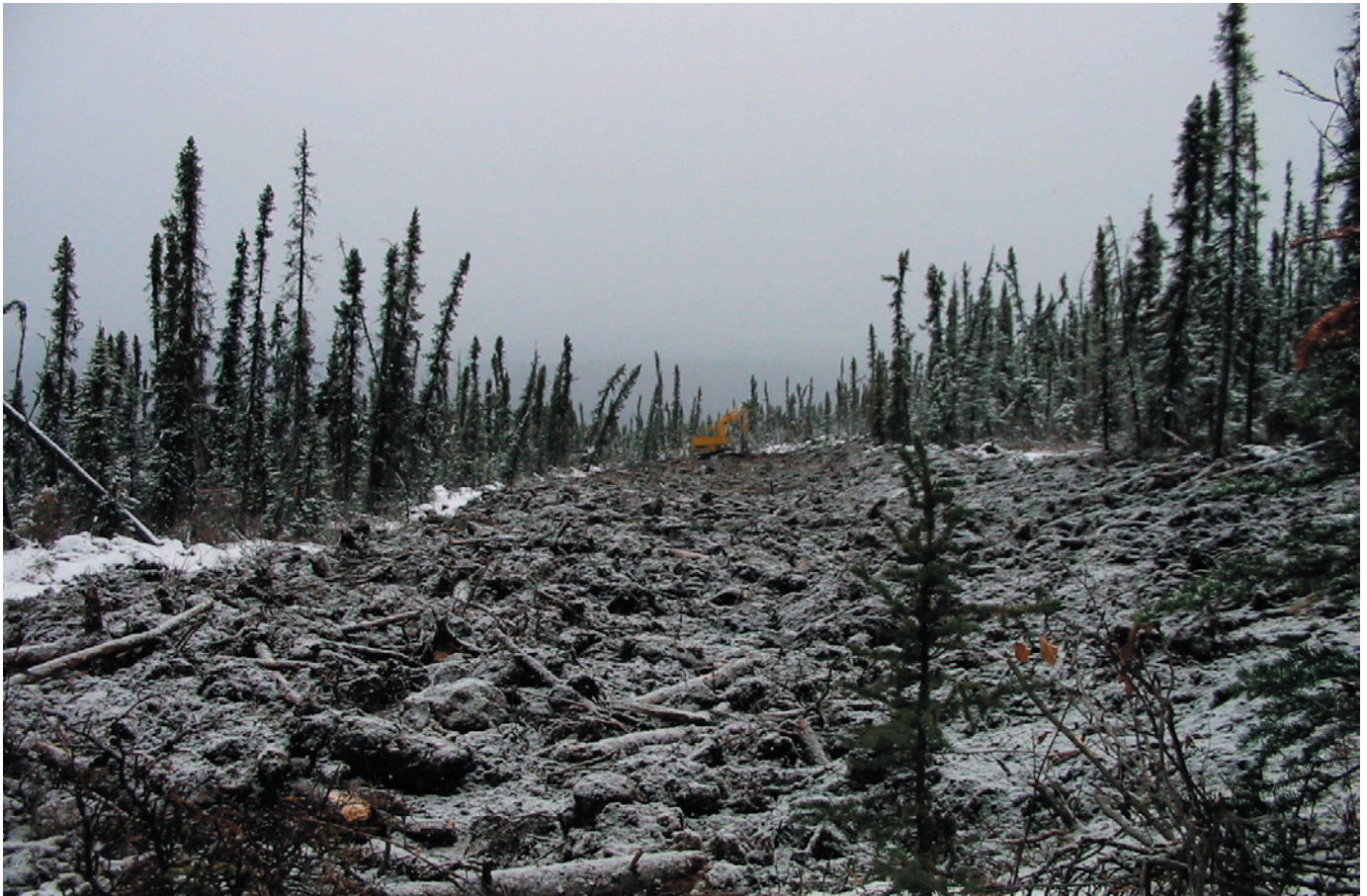
Figure 4. Road reclaimed on the Aurex property using dragback technique, which prohibits access by snowmachines, ATVs and other off-road vehicles.
