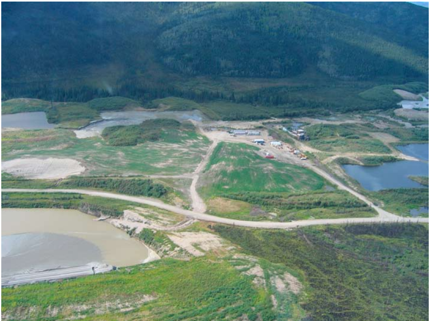
Figure 4. Steep structures have been recontoured to low-relief angles, and vegetation is flourishing from the addition of overburden spread on the surface.
