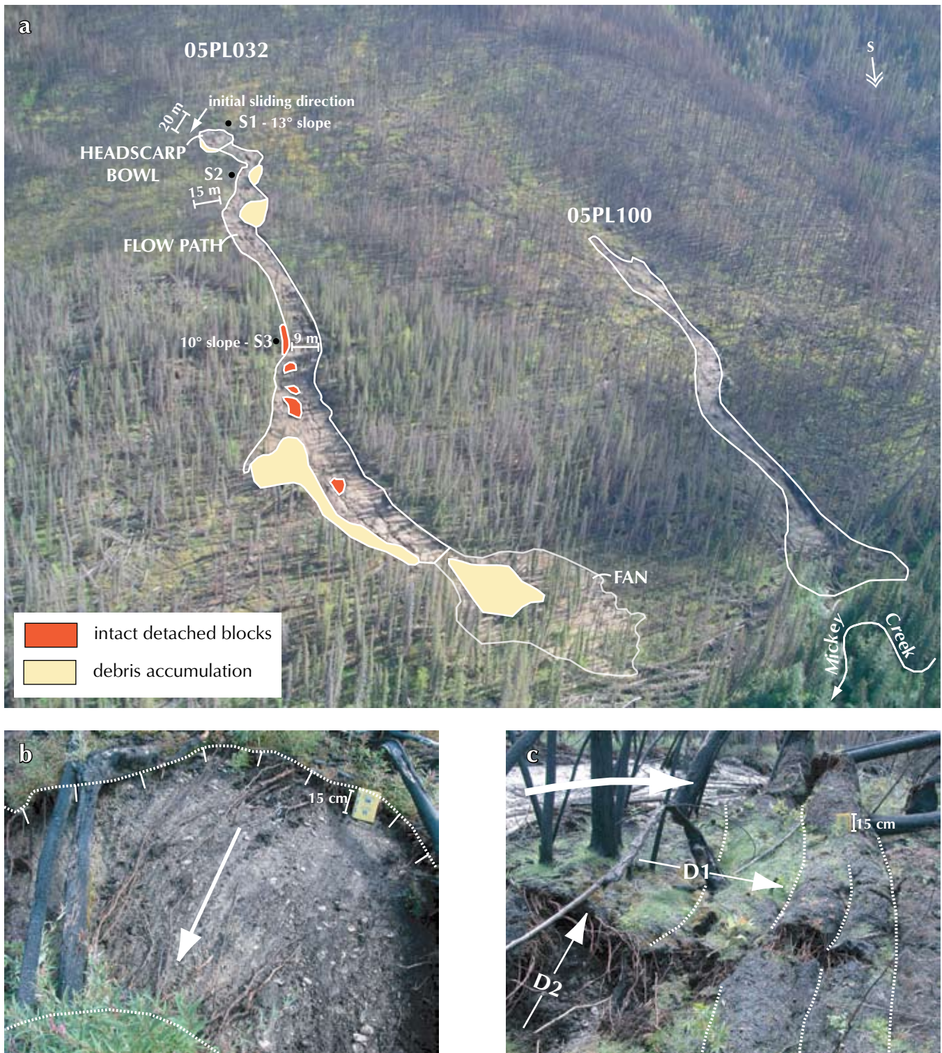
Figure 6. (a) Oblique aerial view of two detachments (05PL032 and 05PL100) that occurred on a gentle south- to southwest-facing slope. The larger failure is over 200 m long and initiated only a few days prior to these photos being taken on July 20, 2005. (b) Detachment of organic mat exposed in tension cracks above the headscarp (location S1 in Figure 6a). Roots are stretched in the direction of sliding. (c) Deformed organic mat (location S3 in Figure 6a), marginal to flow path (heavy arrow). The mat was initially compressed (direction D1) to form folded compression ridges (small dotted lines). It was then torn away from the surrounding mat (direction D2).
