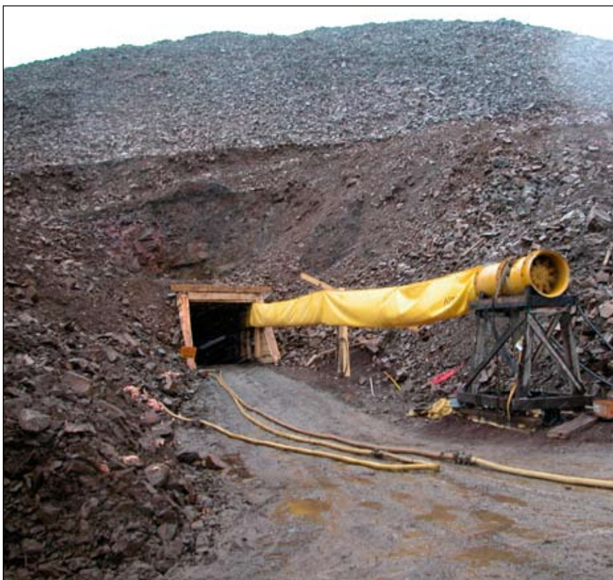
Figure 21. Rehabilitated portal at the MacTung tungsten deposit.
