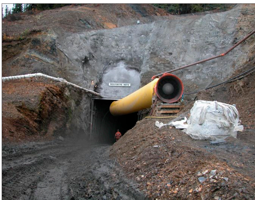
Figure 28. Portal entrance to the Wolverine deposit.
