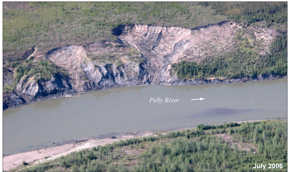
Figure 9. Oblique aerial photograph of a retrogressive thaw slump (#5 in Fig. 3) that was contributing sediment to the Pelly River in 2006. This landslide has been active and increasing in size since at least 1989. View is to the south. Estimated width of main failure is approximately 200 m.
