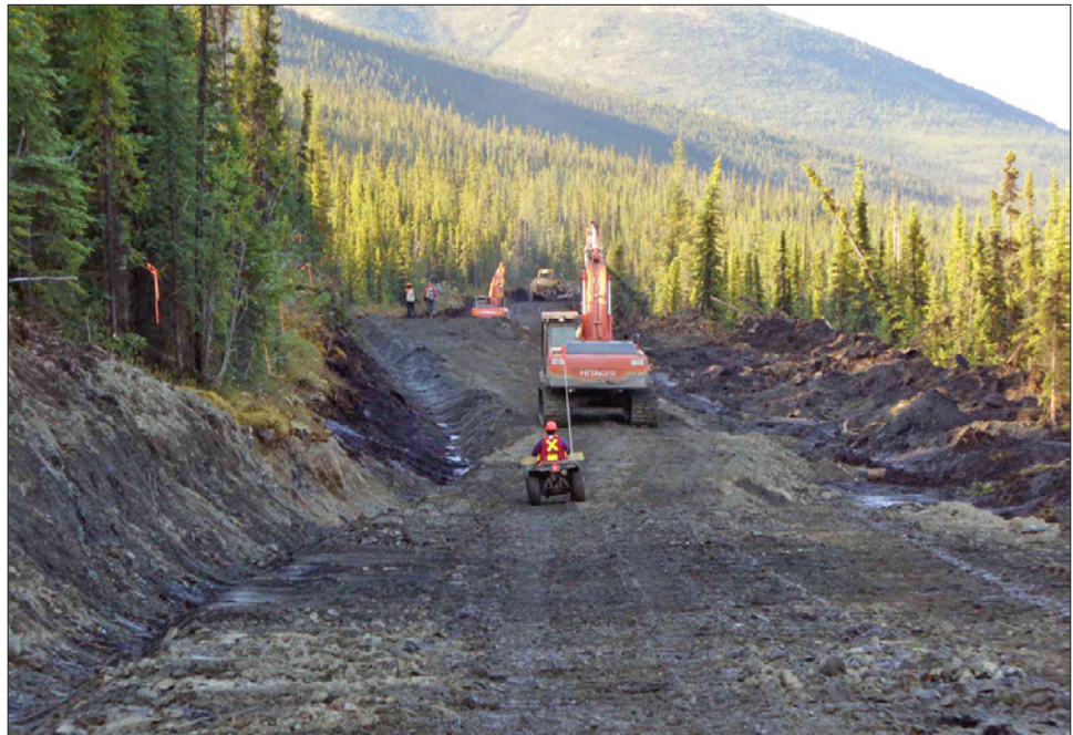
Figure 7. Wolverine mine access road development. Photo by Yukon Zinc Corp.
