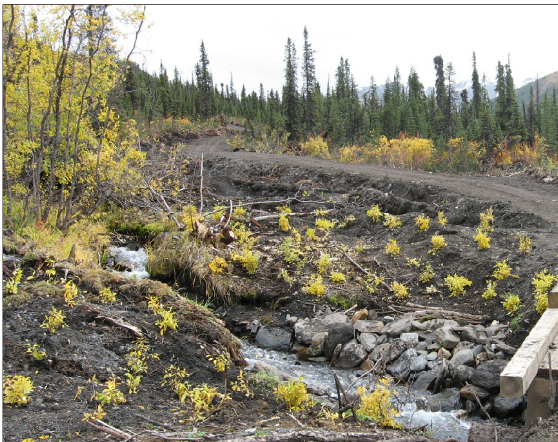
Figure 1. Bio-engineering in the Don Valley: live willows are being planted to stabilize the banks of the road.
