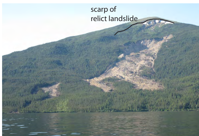
Figure 2. View of the Little Salmon Lake landslide.
