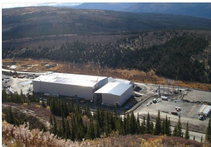
Figure 8. Wolverine mill building under construction. (Photo credit: Yukon Zinc)
