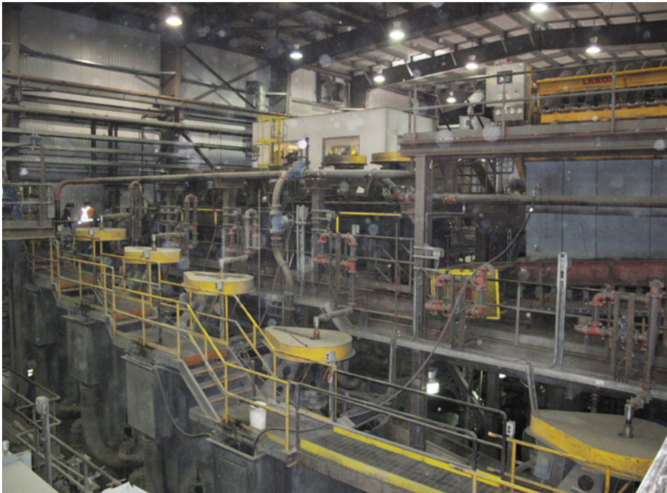
Figure 6. The Minto mill building.
