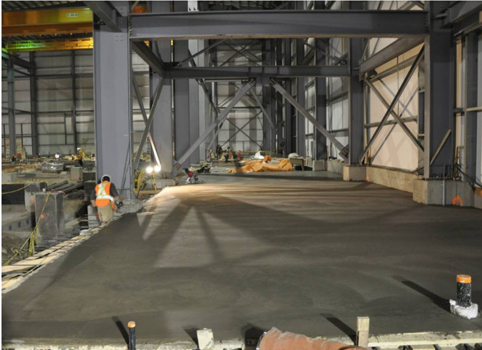
Figure 9. Construction inside the Wolverine mill building. (Photo credit: Yukon Zinc)
