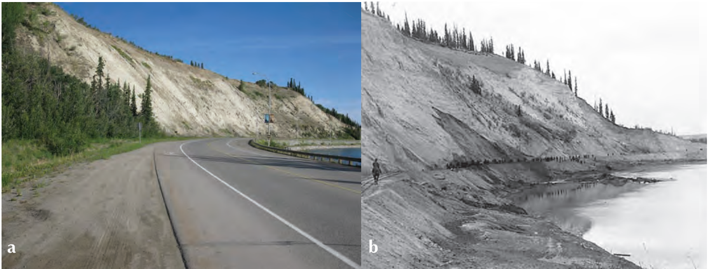
Figure 2. (a) View of a silt bluff at the southern end of town along Robert Service Way, where the road is confined between the base of the bluff and the Yukon River; (b) photo taken at the same location, ca. 1900, where a minor landslide was being cleared from the railroad track (historical photo by H.C. Barley Fonds from the Yukon Archives, #5416).
