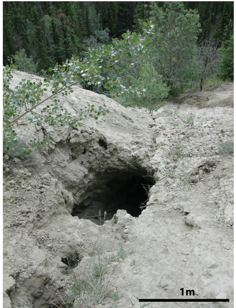
Figure 23. Photo of piping erosion observed at station MAB 09-17-02.
