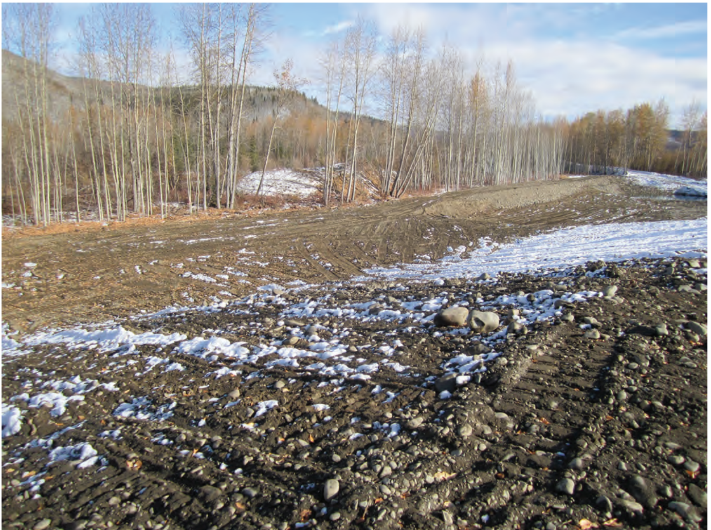
Figure 3. Berm/trail created to alleviate flooding.
