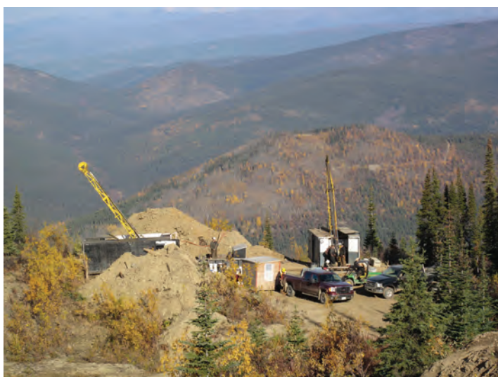
Figure 22. Geotechnical drilling at the Eagle Zone, Dublin Gulch property.
