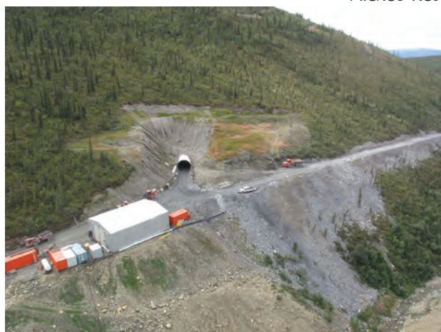
Figure 8. Portal at Bellekeno Mine.
