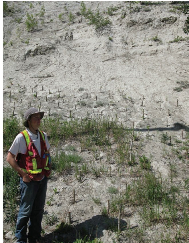
Figure 24. Examples of the remediation effort completed to reduce erosion of the bluffs in downtown Whitehorse: (a) check dam to reduce flow velocity and encourage deposition; and (b) planting of grass and tree saplings in order to reduce erosion due to overland flow, and to increase soil strength by increasing the root network.
