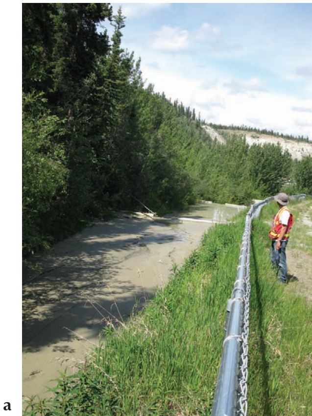
Figure 24. Examples of the remediation effort completed to reduce erosion of the bluffs in downtown Whitehorse: (a) check dam to reduce flow velocity and encourage deposition; and (b) planting of grass and tree saplings in order to reduce erosion due to overland flow, and to increase soil strength by increasing the root network.
