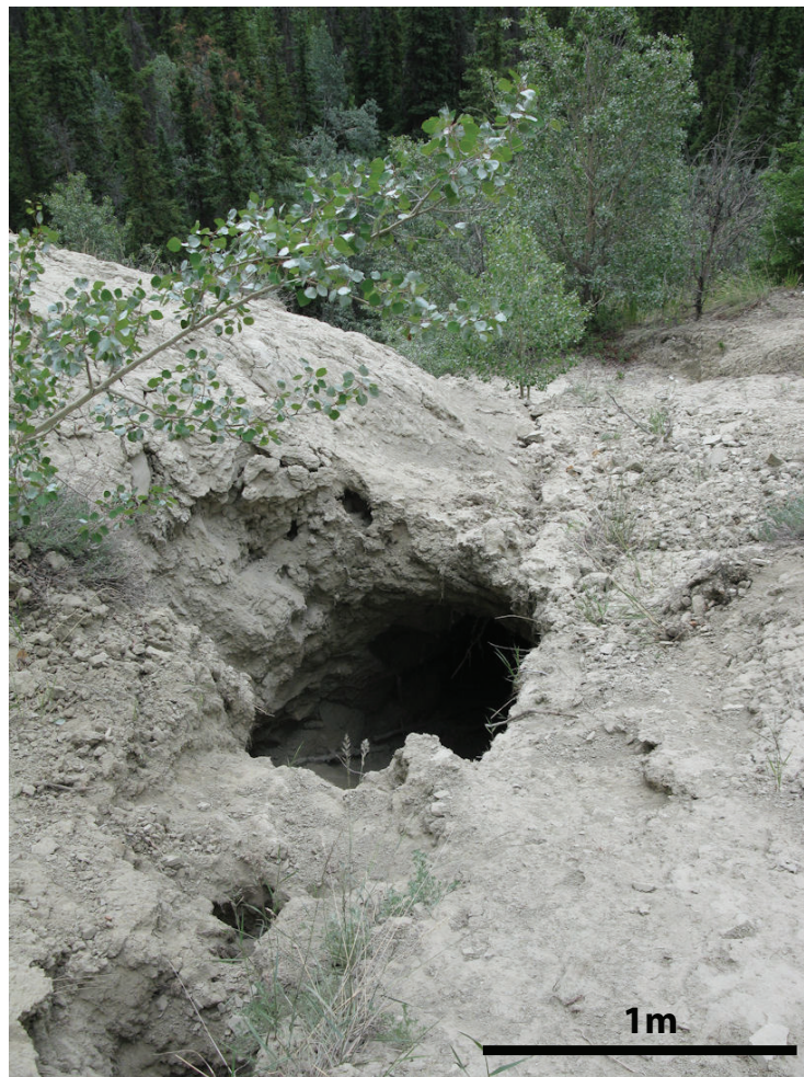
Figure 23. Photo of piping erosion observed at station MAB 09-17-02.
