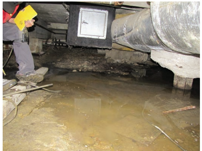
Figure 5. Water in crawl space beneath Palace Grand Theatre, July 25, 2010; note the exposed piling below concrete pad indicating the presence of ground surface subsidence.
