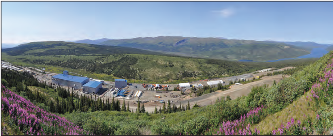
Figure 1. Yukon Zinc's Wolverine mine site, July 2010.
