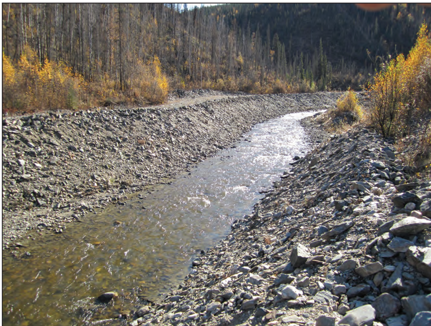
Figure 2. Stabilized creek channel.
