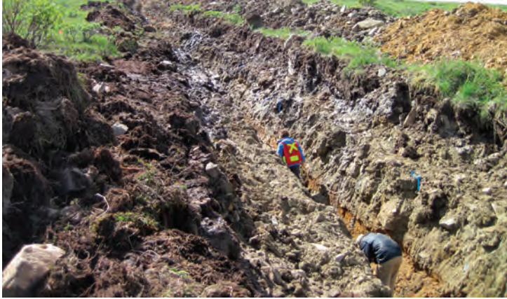
Figure 25. Rockhaven Resources' impressive trench at the Klaza property.
