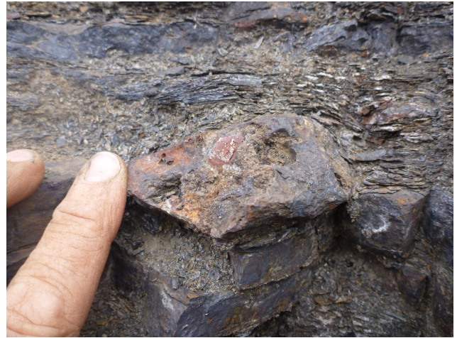
Figure 15. Highly weathered ammonite nodule, now replaced with pyrite, which has preferentially weathered out leaving holes in the nodule.
