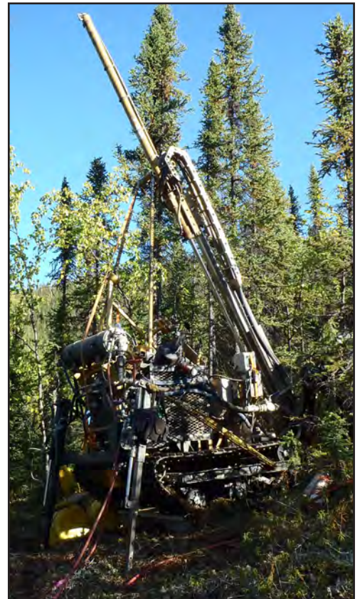
The RAB, a lightweight drilling rig, on-site.
