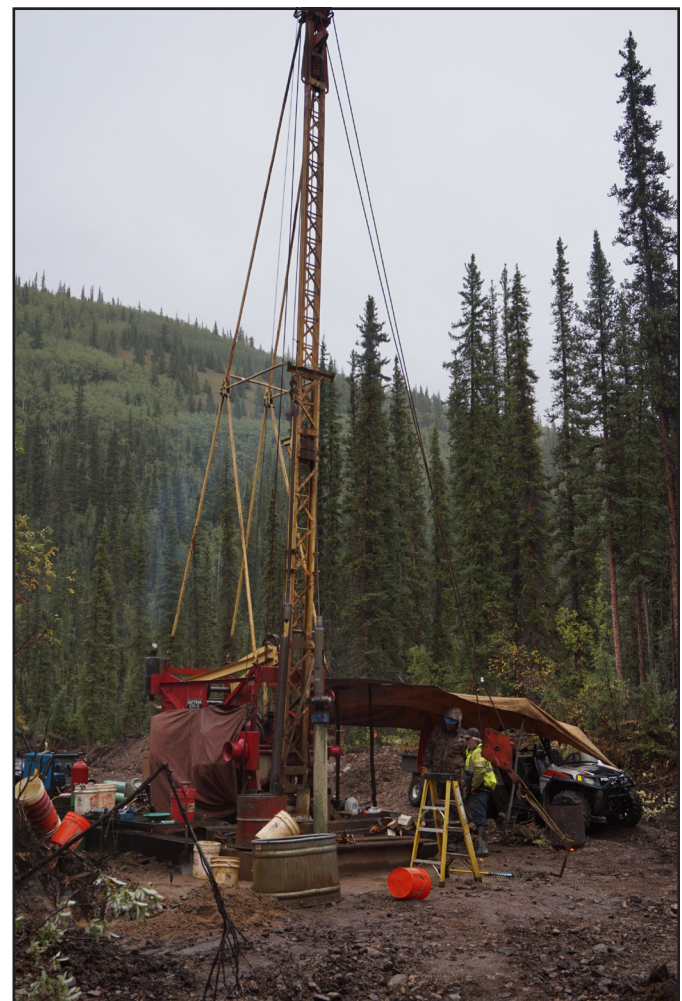
Figure 14. A view of Derek Dodge’s refurbished 1950s-vintage cable tool rig on Seymour Creek. Drilling the 6” cased holes was slow (5-7 days per hole), but was able to accurately delineate a channel at approximately 27 m (90 ft) depth. The rig was also able to sample the pay zone in 30 cm (1 ft) intervals helping to define the gold distribution.
