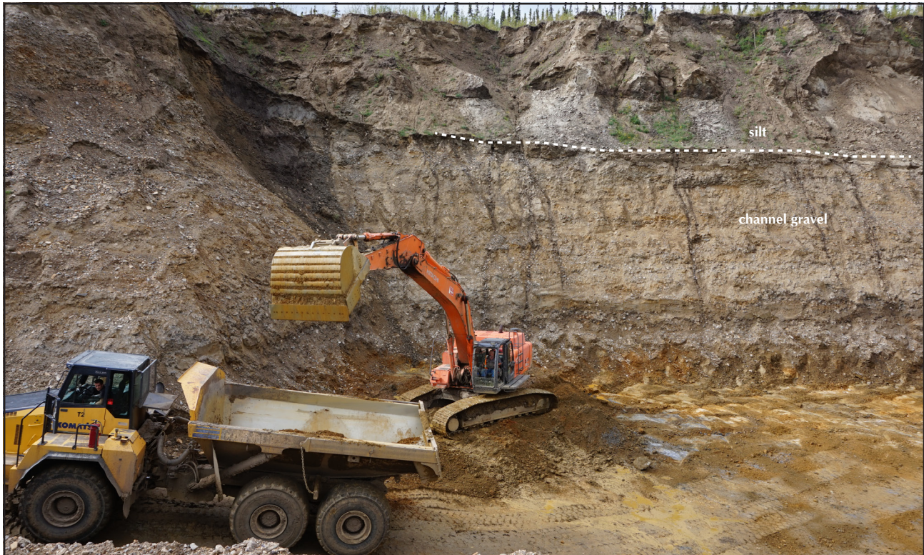
Figure 3. View of Fine Gold Resources 2015 pit on the left limit bench channel of Eureka Creek. The cut consists of 16.5 m (54 ft) of gravel overlain by 9 m (30 ft) of silt (loess). Both units are frozen. The bedrock surface continues to dip into the face and the full width of the channel has not been exposed.
