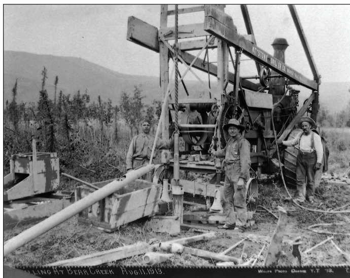
Figure 3. Keystone churn drill active on Bear Creek in 1913 (Wolfe, 1913).
