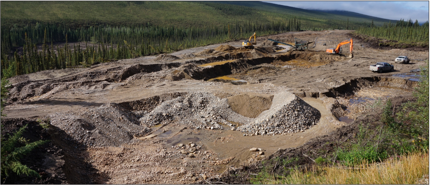
Figure 14. M2 Gold's operation on the 60 Mile River bench in 2016. A 50 m-wide cut was processed along the rim of the bench using two excavators and a mobile plant.
