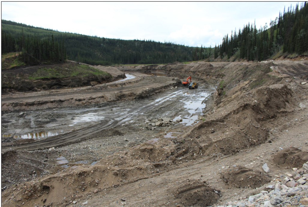
Figure 11. H.C. Mining operation on lower Henderson Creek in 2016.
