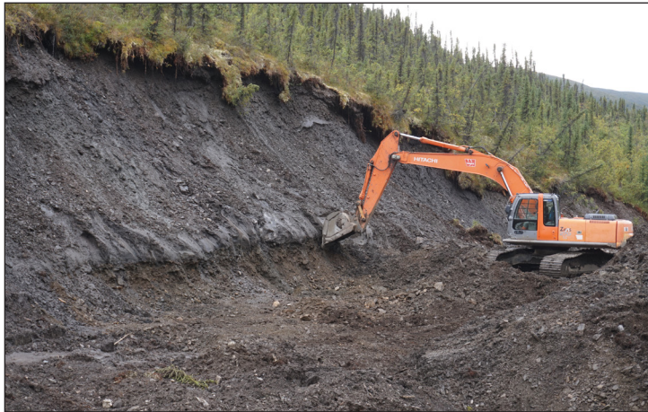
Figure 15. A view of the right limit bank on upper Glacier Creek. K-1 Mining is excavating the pay streak under colluviated weathered bedrock and muck.
