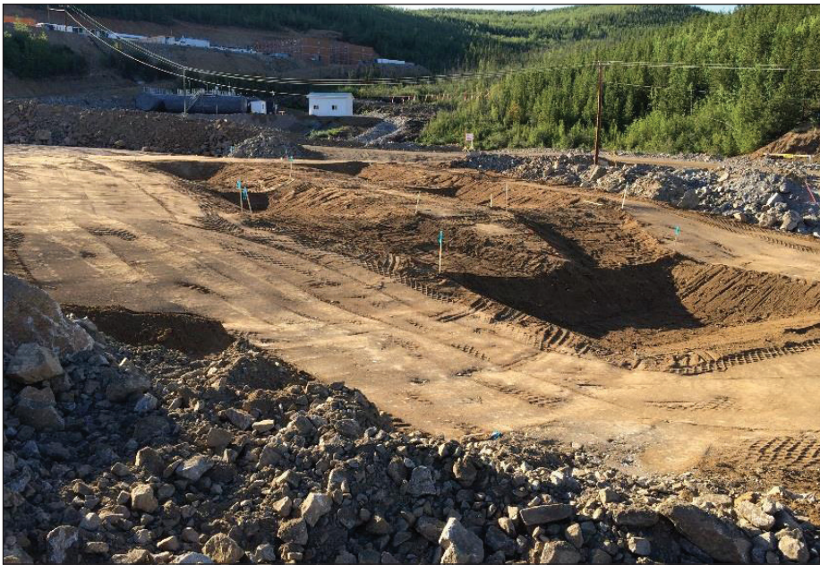
Demonstration scale CTWS foundation during construction.
