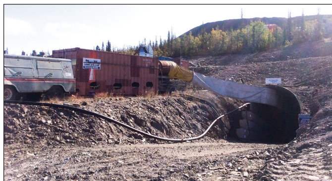
Figure 6. Bermingham mine portal.
