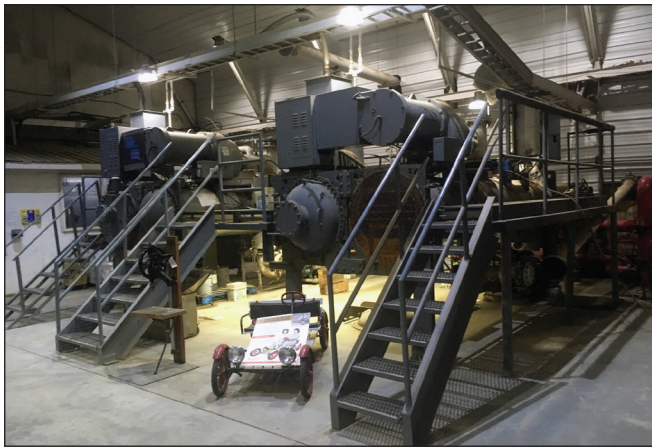
Figure 16. Two binary-system power plants generate 0.4 MW of electricity at the Chena geothermal plant.
