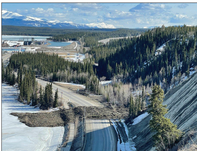
Figure 6. View looking south along Robert Service Way (Whitehorse) at debris from an April 30th 2022 landslide that closed the road for several weeks.
