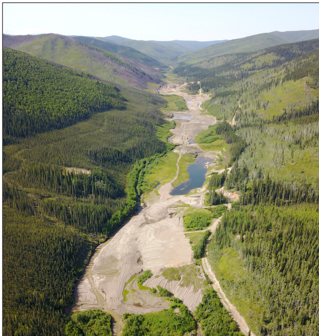
Figure 12. Reclamation on lower Maisy May Creek completed by Bedrock Mining Company Inc. this season. The view is looking upstream.
